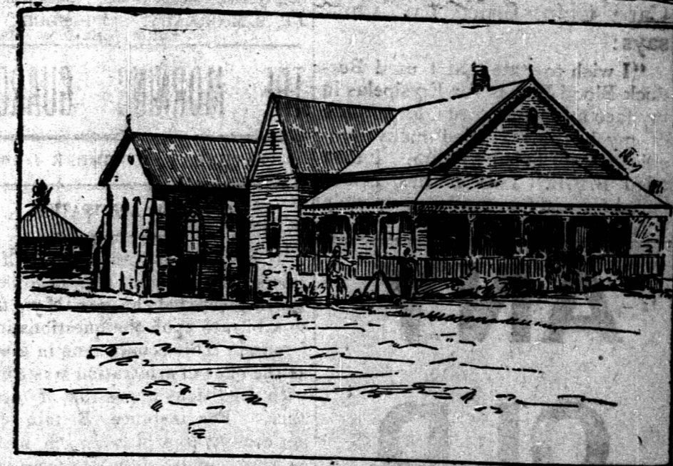
CHURCH AND PARSONAGE TYPICAL OF THE TRANSVAAL
