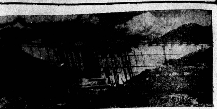
NEARLY FINISHED - Giant Shasta Dam in California is almost completed, with mass concrete placement scheduled to end early in July. Shasta Lake already contains more than 975,000 acre-feet of water awaiting completion of control gates before starting downward plunge.
