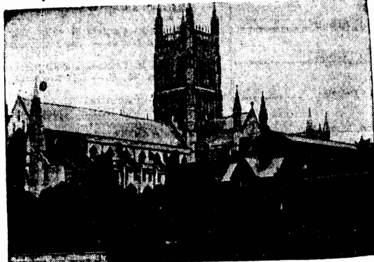
Canon E. F. Braley has ordered a stop to bellringing in the central tower of 865-year-old English Worcester cathedral when caretakers found two 40-ton pinnacles on the tower badly cracked and in danger of falling. The canon was afraid vibration from the bells would jar the huge pieces of masonry off their piers. Repairmen estimated it will take two months to make the pillars of one of the loveliest churches in England secure and cost will be about $80,000. Braley, who is worried about how "to come by the money," told reporters that "All the lipstick and face powder of the tower, as it were, has deteriorated."
