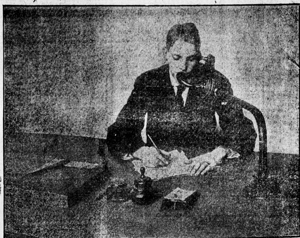
DISPATCHING TRAINS BY TELEPHONE ON THE C. P. R.
