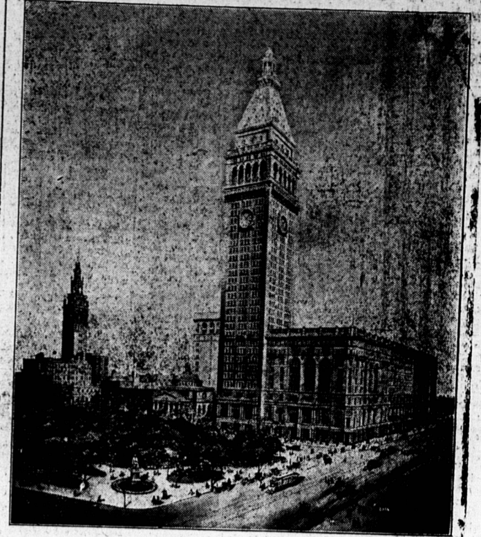
Metropolitan Life Building, New York City, the Tallest in the World.
