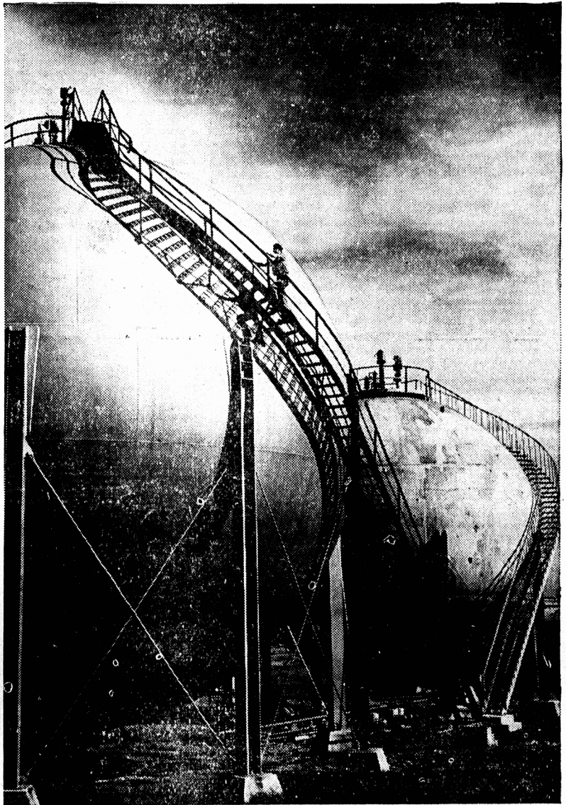
Hortonspheres at Shell Oil plant are slightly different from Imperial's. These contain normal butene and butane butylene used in making 100-octane gasoline for aviation. Ordinary car gas was reduced from 80 to 74-76 octane as a war measure.
