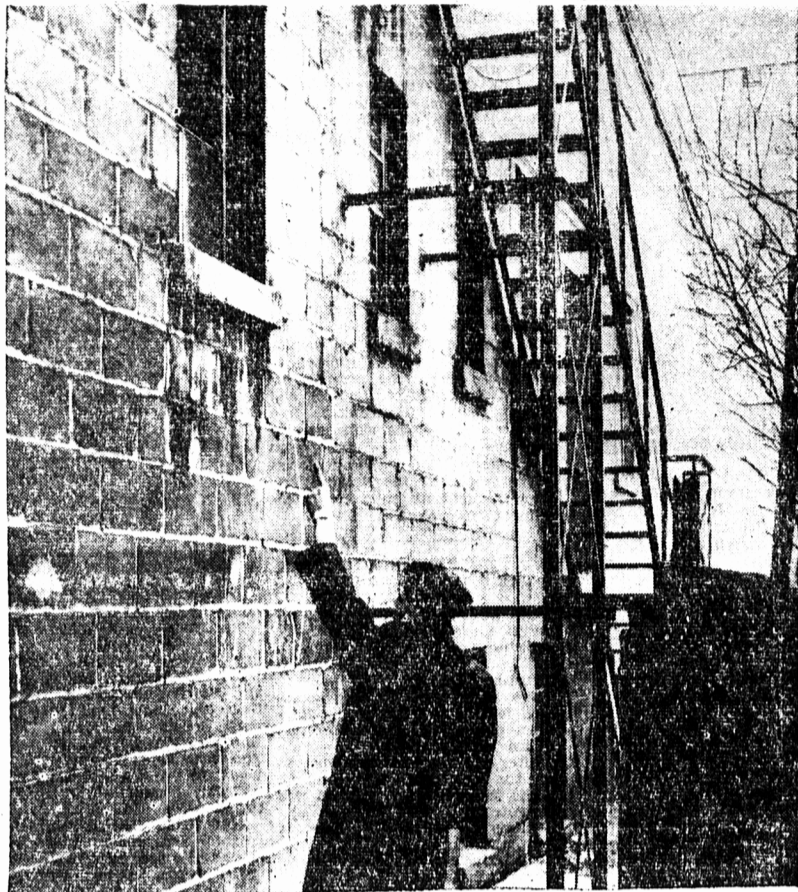
Six persons died in the flames set off in the basement of a clothing factory in Toronto when the boiler exploded. At least seven others were trapped behind barred windows until firemen cut their way to them with acetylene torches...
