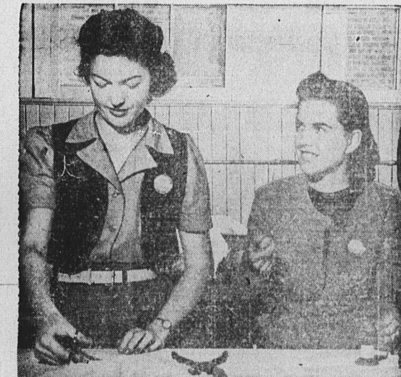
Canadian girls are shown ABOVE at work on the fabrics of the Norseman wings. These girls are doing their share in providing wings for the training of empire fledglings. A plant supervisor is shown in the background inspecting the work of a girl sewing kapok, used as insulation against cold, heat and sound in Norseman "flying classrooms."
