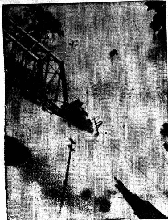
Three train crewmen escaped death by swimming to safety when this Pennsylvania Railroad engine crashed into Lycoming creek near Williamsport, Pa. Flood waters weakened approach to the bridge.
