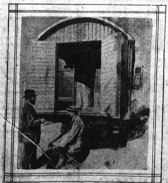
RESERVOIR HOUSE USED BY ENGINEERS
