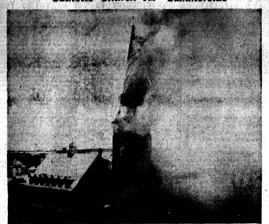
The above picture of St. Paul's Roman Catholic Church, Summerside, was taken about 11 o'clock Sunday morning, just as it was becoming apparent that firemen were losing their battle to save the 70-year-old brick and wood structure from destruction by fire. Both these pictures were taken from the Summerside Court House cupola.
